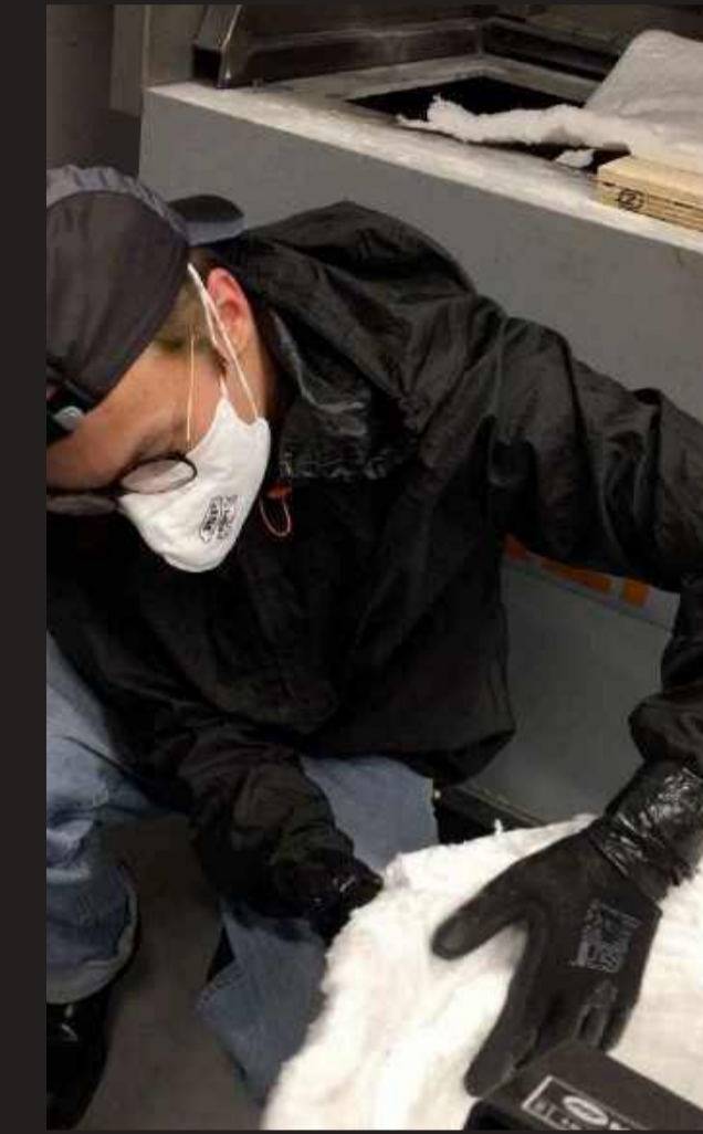
6-The wires are put through to hold the fire blanket.
