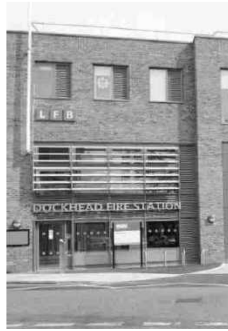
7. Dockhead Fire station
