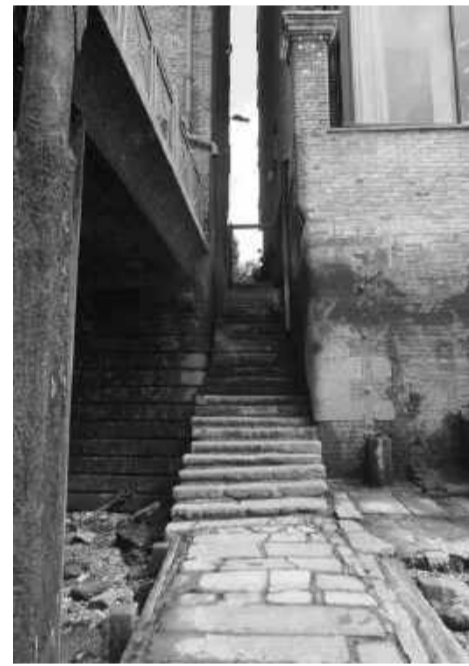
2. Alderman Stairs and Gate Piers
