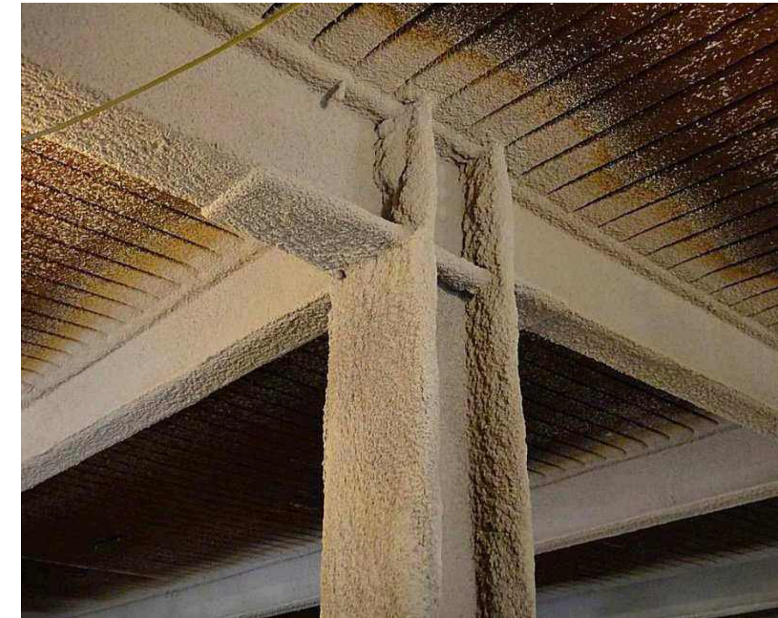
Replacing fire coating insulation with clay instead of concrete.
