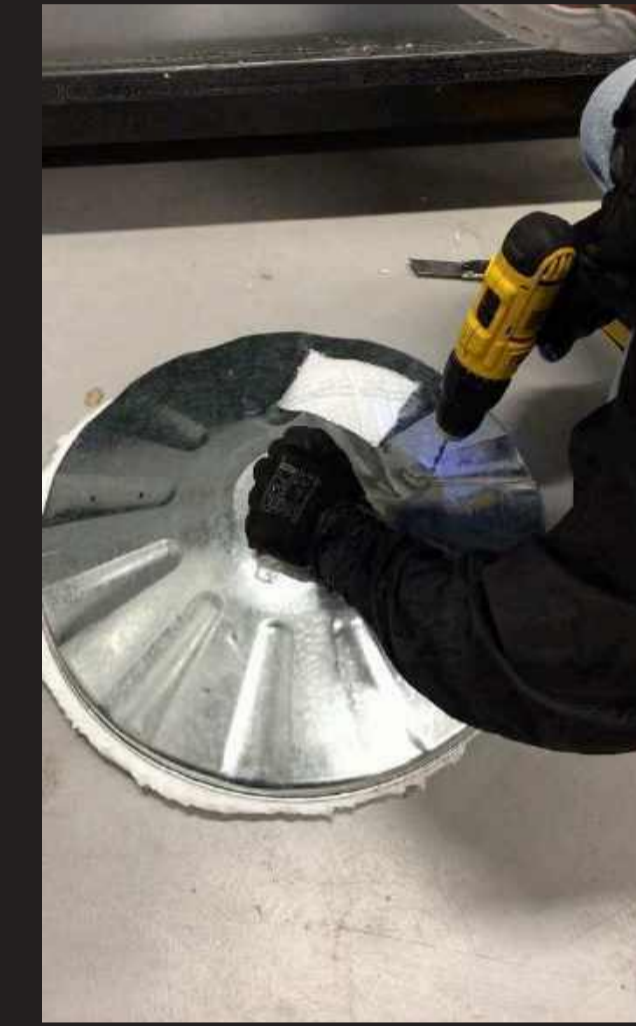
5-Holes are made for fire resistant wires.
